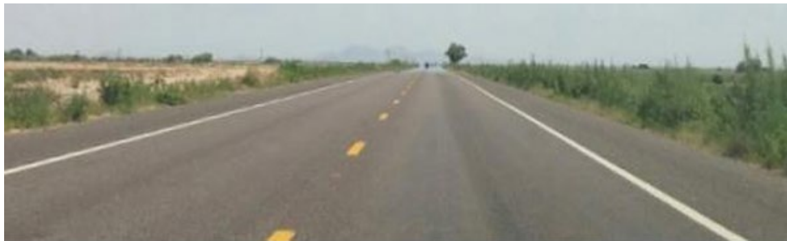
Example of a roadway with good pavement condition
